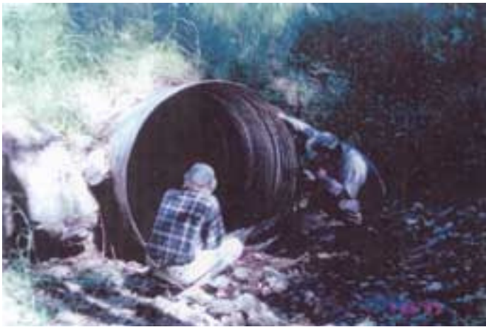
View of new culvert inlet, 07/26/99
