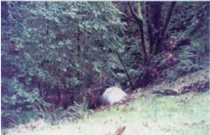
Outlet with downspout, 01/10/01
