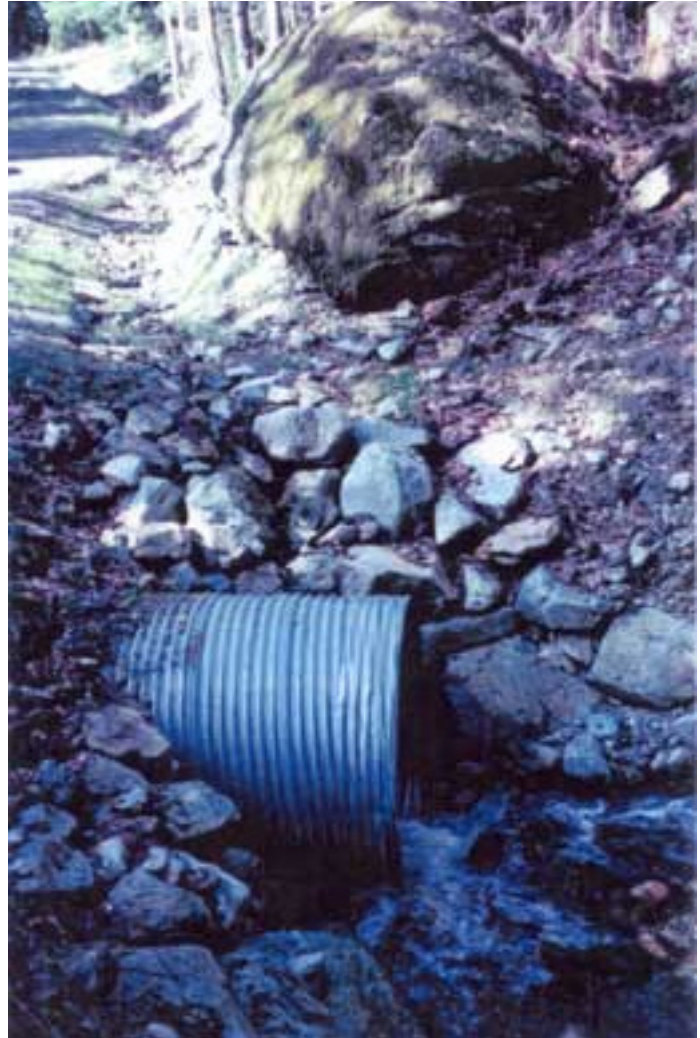
View of armored inlet, ditch runoff into inlet basin, 04/06/99
