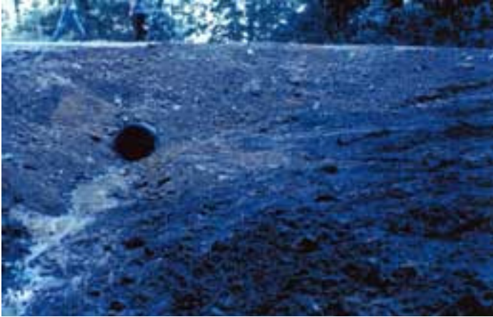
Inlet after installation, 09/17/99
