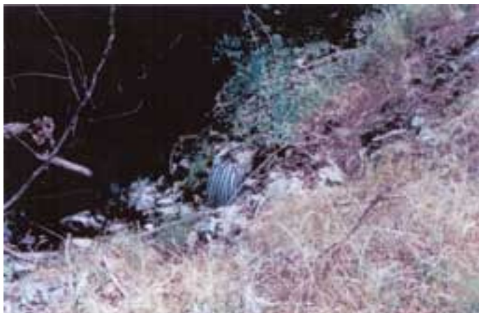
Outlet on rock, 07/26/99
