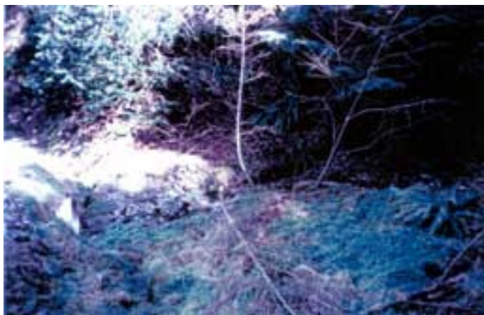
Deposit upstream of inlet with headcut, view from side, 04/06/99
