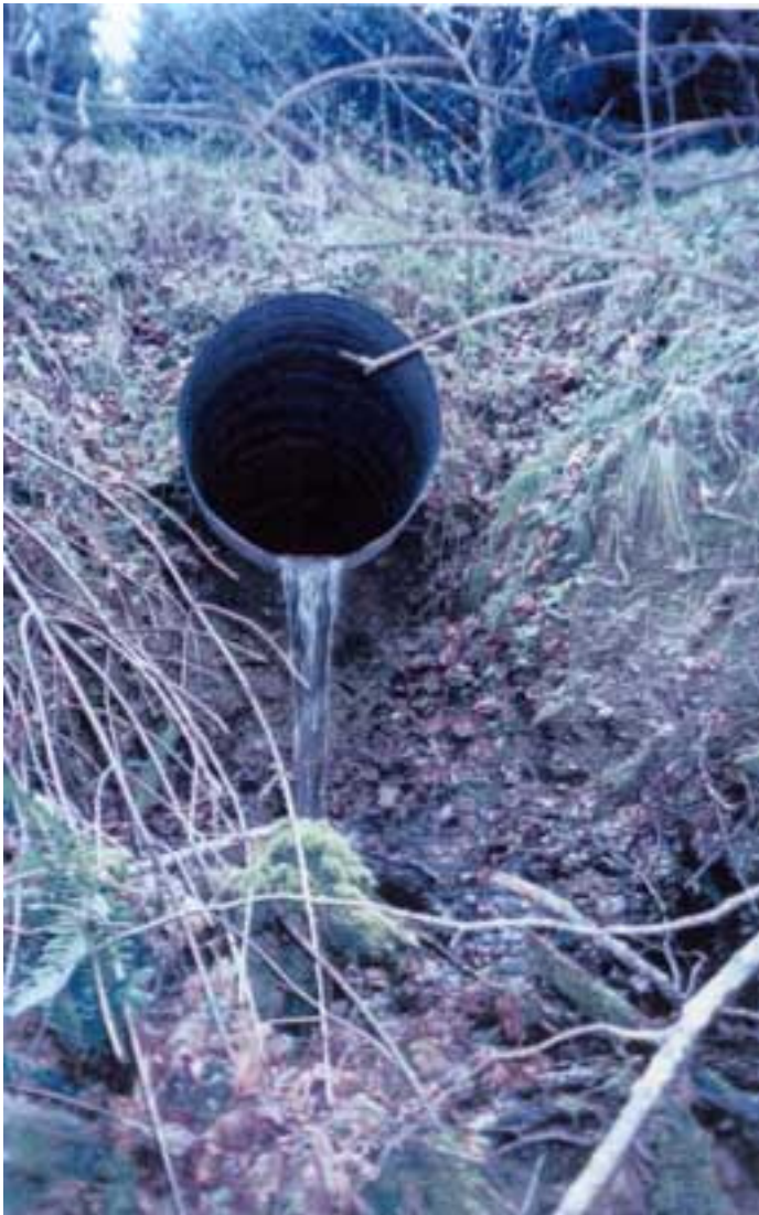
Outlet view from downstream, small rills on fill, 01/10/01 Inlet with rusting invert and substrate deposit, 01/10/01
