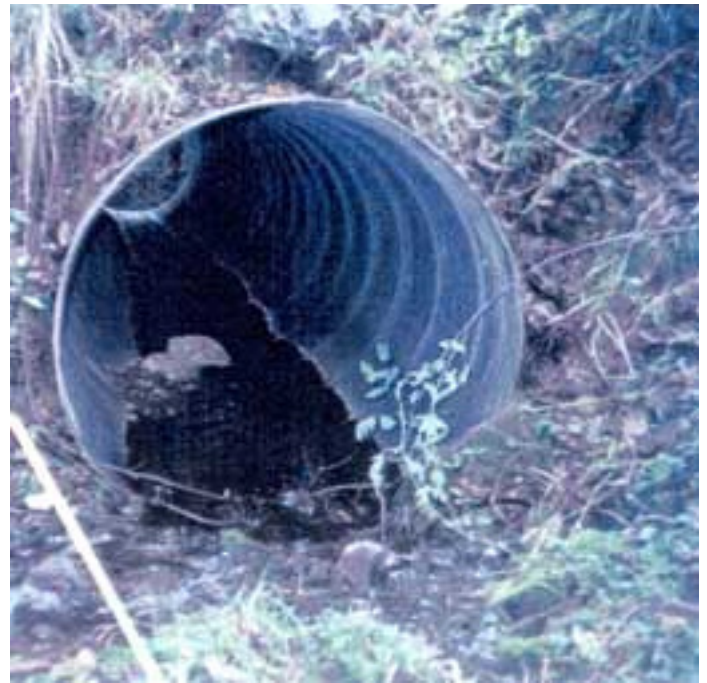
Outlet view from downstream, small rills on fill, 01/10/01 Inlet with rusting invert and substrate deposit, 01/10/01
