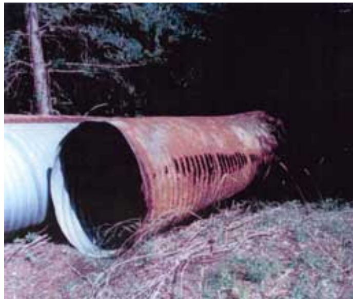
Pipe that was replaced
