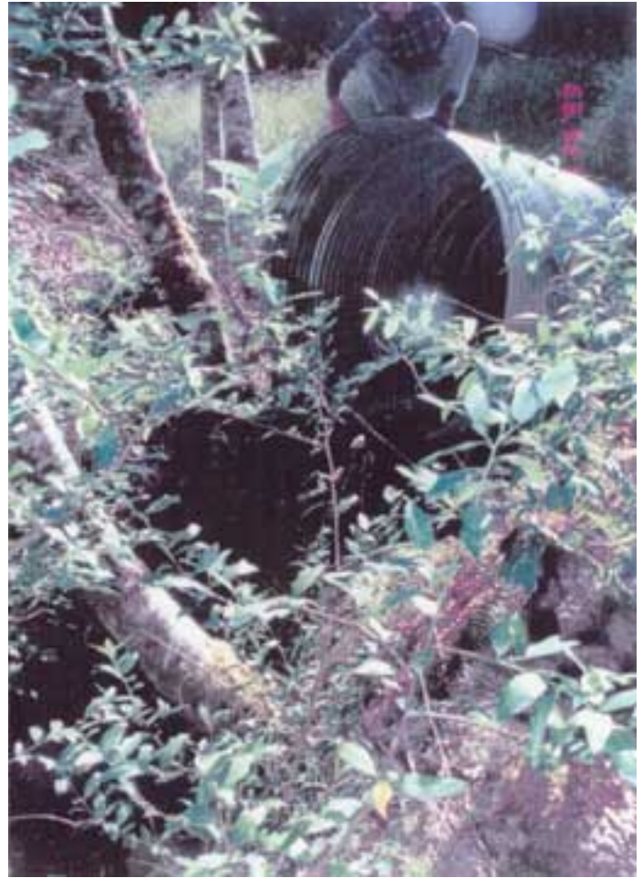
View of new culvert outlet, 07/26/99
