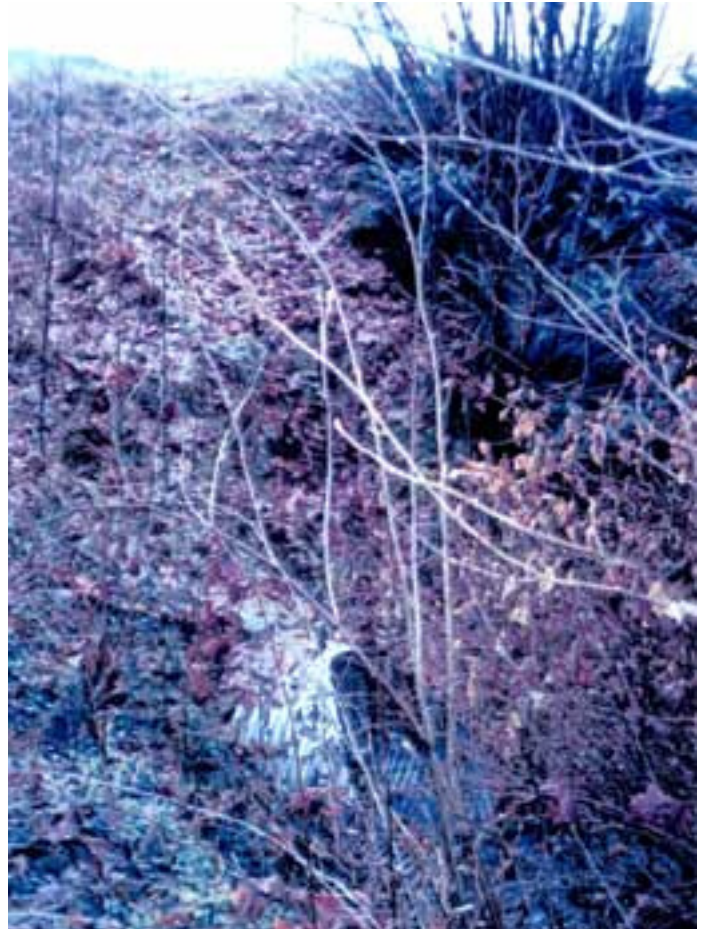
Inlet view note alders in foreground, 01/10/01
