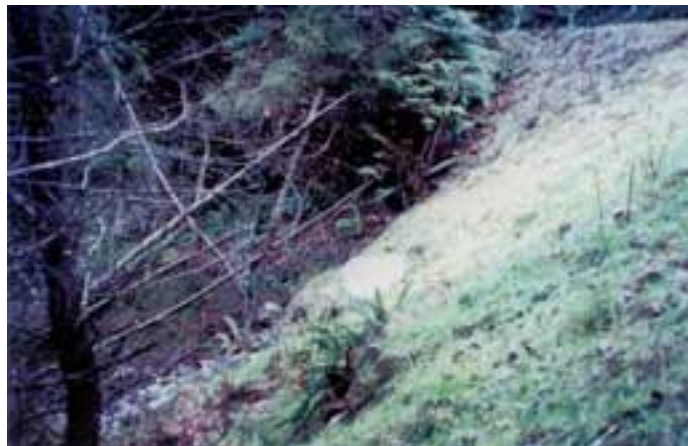
Outlet, note stable bank, 01/10/01
