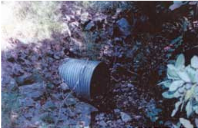
48" pipe, inlet on rock, 07/26/99
