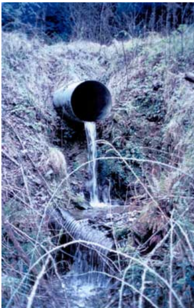
Old pipe creating step in channel, preventing downcutting 01/10/01 Headcut stabilized, view upstream, 01/10/01.
